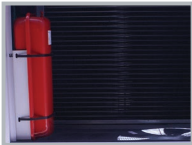
closed expansion tank
